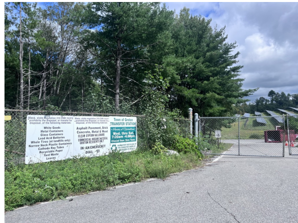
Groton Transfer Station
